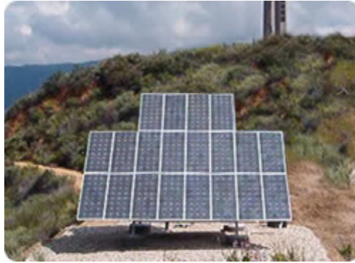
This 2400W Power Station is used to power a Microwave Repeater Site.
