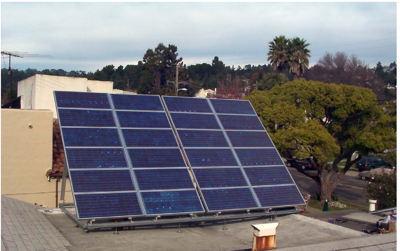
PV Installation utilizing the Grid-Beam Spaceframe for uneven roof surfaces.
