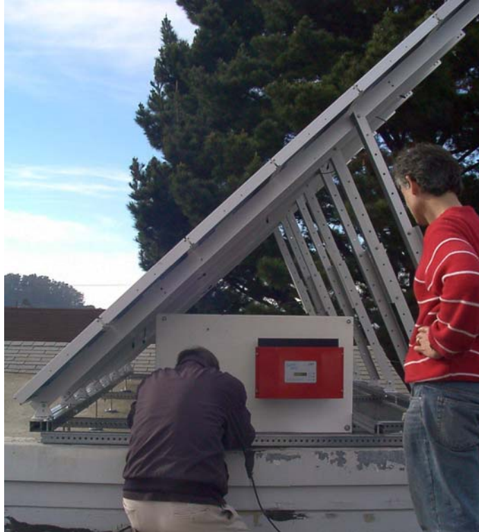
Sunnyboy UT 1100SB PV Installation directly to the Grid.
