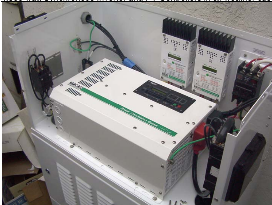
4,800 watt Synchronous Inverter and PV Controllers in all weather case
